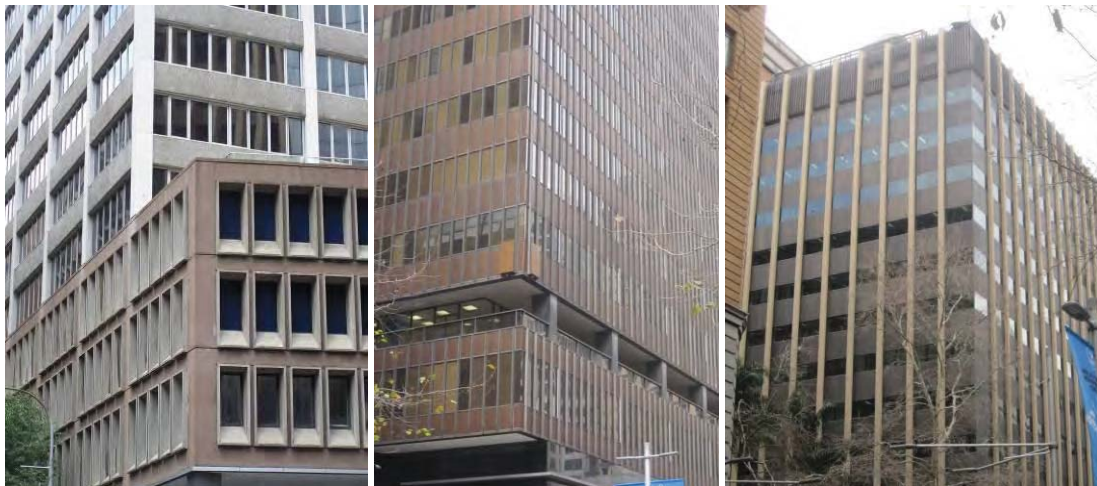
Figure 36 ANZ Bank, 29 Hunter Street, showing the differing treatment of podium and tower fenestration (left), ES&A Bank, 18-20 Martin Place (centre) and Bank of New Zealand, 4-6 Wynyard Street (right). The ES&A and Bank of New Zealand buildings both show the persistence of the curtain wall in the late 1960s and early 1970s, and the subtle way its aesthetic changed.
