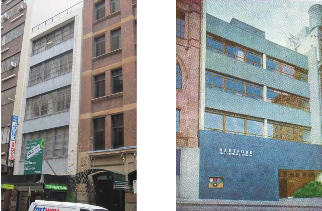
Figure 18 36 York Street (left) and 48 Margaret Street (right). Their external design and claddings harken back to the pre-war period. The exterior of 36 York Street is clad in dichromatic terracotta, while the ground floor of 48 Margaret Street was clad in dark toned ceramic tiles and the horizontal upper sections in light-toned porcelain enamel steel. The small garden at the main entrance to 48 Margaret Street was an innovative feature. Sources: TKDA (36 York Street); Architecture , April-June 1954, p.85 (48 Margaret Street).
