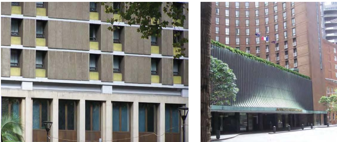
Figure 71 The rational precast concrete facade detailing of Menzies' Hotel (left) contrasts with the dramatic sweep of the light court and canopy of the Wentworth Hotel (right). Source: Roy Lumby.
