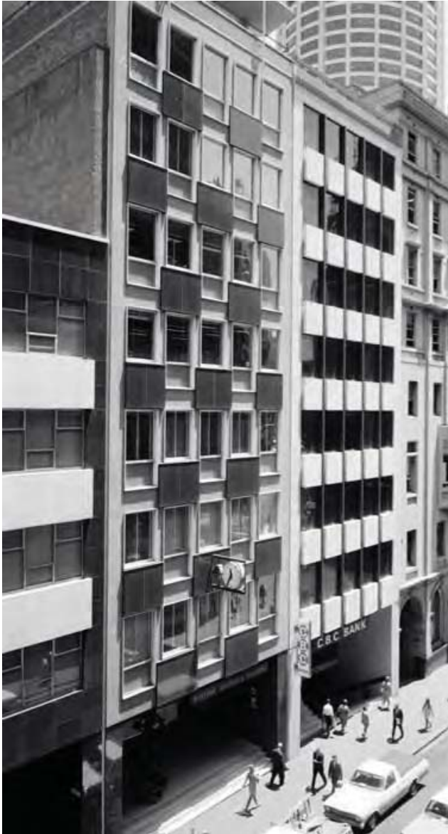
Figure 24 The 3 buildings at 105-113 Pitt Street demonstrate the tendency towards masonry and precast claddings during the 1960s: the base of 109-113 Pitt Street, designed in 1960 by Rudder Littlemore & Rudder (left), 107 Pitt Street, designed for Western Assurance by McConnel Smith & Johnson in 1958 (centre) and 105 Pitt Street, designed for the Commonwealth Bank by J A & P Kerr in 1965/66 (right). Source: NAA image no. A1200, L79768.
